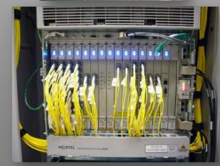
Multimode 62:5/125 (OM1) Datacomms \*Multimode 50/125 (OM2) Video & Datacomms Systems \*Multimode 50/125 (OM3) Gigabit Ethernet and 10 Gig Ethernet for up to 300m \*Singlemode 9/125 (OS1) Gigabit Ethernet and 10 Gig Ethernet for up to 2km.
